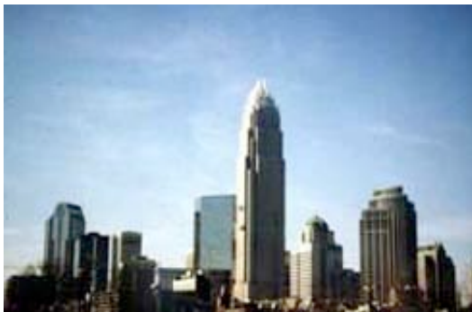
Downtown Charlotte, NC. Note the steep rent gradient implied by the height of buildings. Click on the image to enlarge. Photo by David Hartgen
