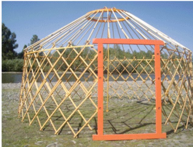
Assembled wood frame
